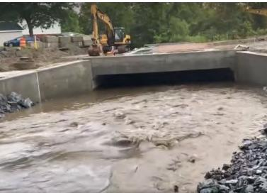
The recently installed box culvert beneath Densmore Drive, shown before and after severe thunderstorms brought drenching rains to town on July 20th, providing this stormwater drainage system its first real test.
